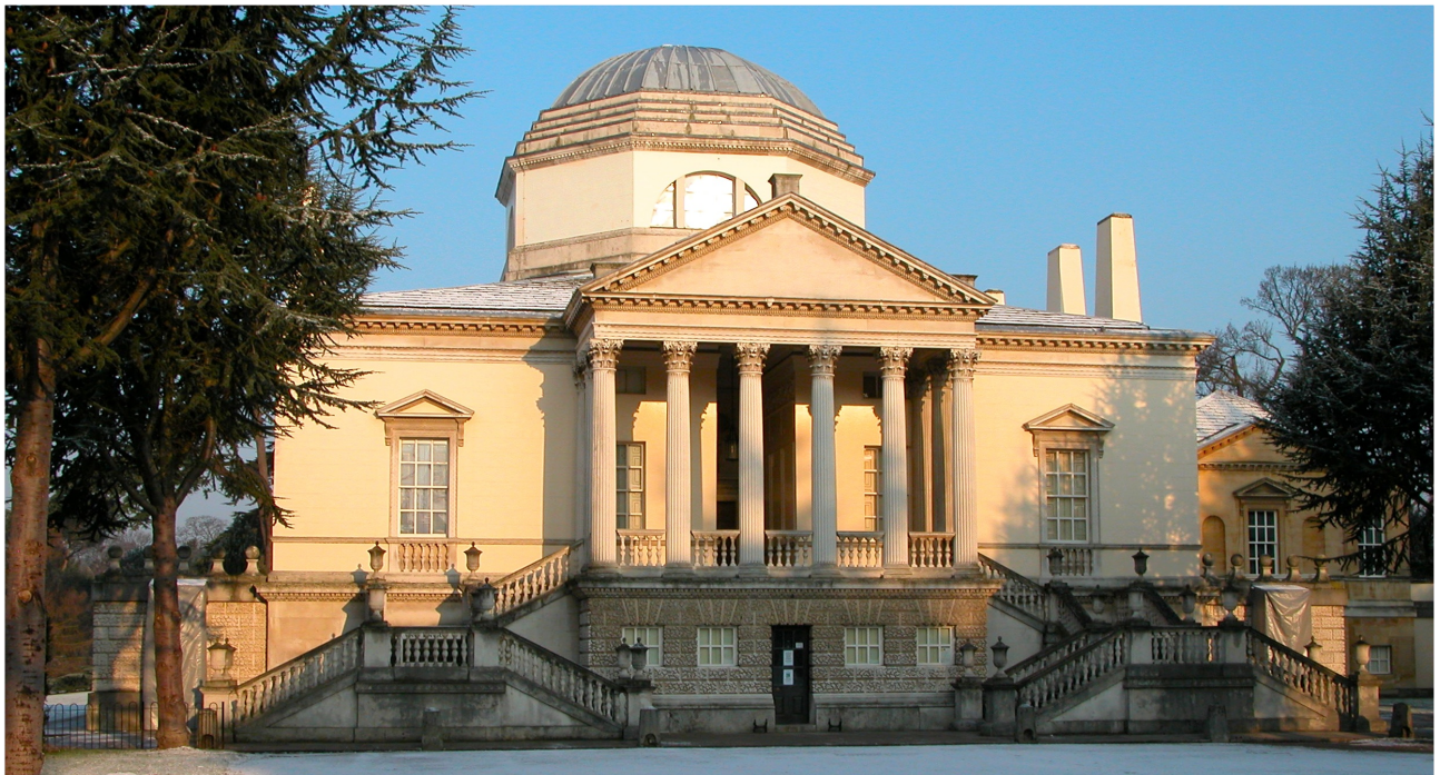
Chiswick House will soon be coated in frost
